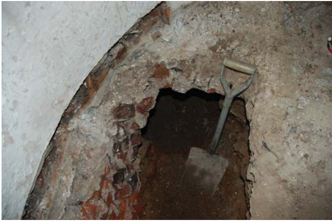
The remains of the seventeenth-century well that was discovered during excavations to the base of the lift shaft. Photograph: John Bridges
