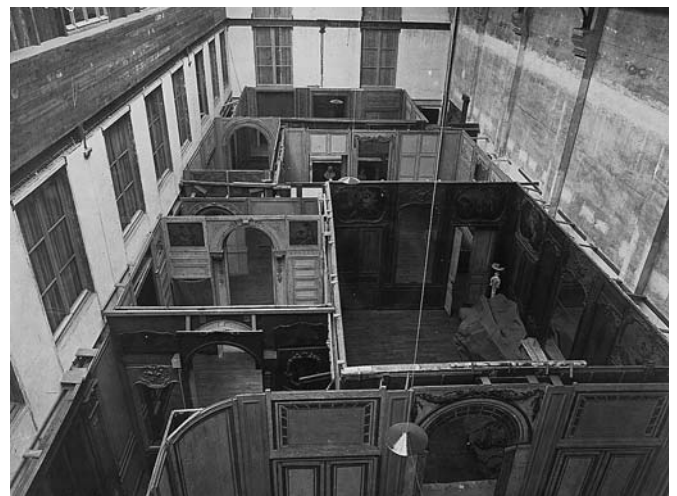
The Knightsbridge Rooms at Roberson's London Warehouse
